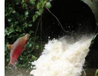
On-Call Hydraulic Services, Fish Passages Improvements WSDOT
